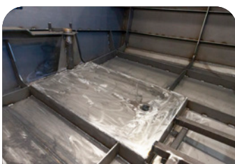
Power Impact Construction (PIC)
