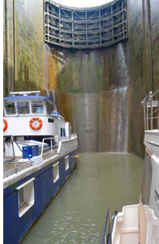
The Bollène lock with a drop of 22 m
