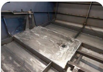
Power Impact Construction (PIC)
